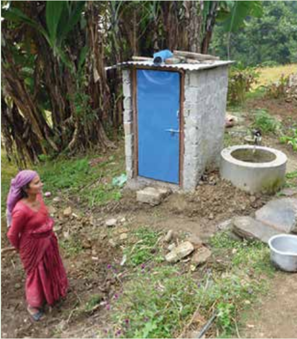
Biogas system connected to a toilet. Photos by the author
