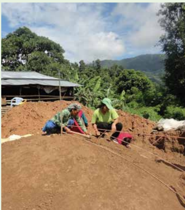
Female biogas masons at work
