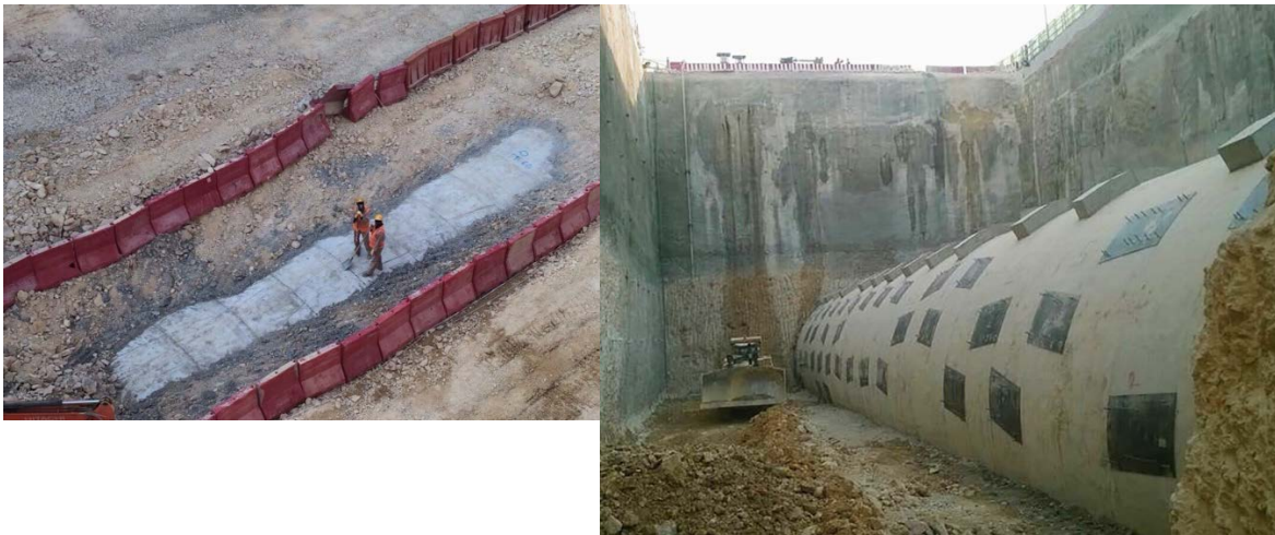
Figure 10. Tunnel crown and lateral excavation with the joints already strengthened
