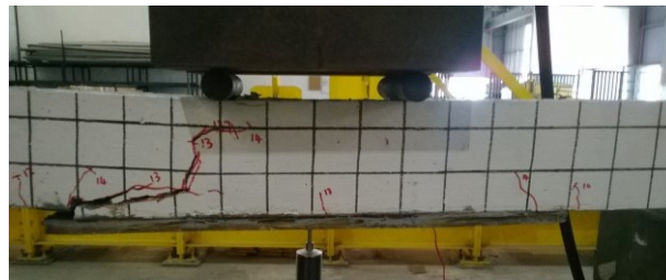
Figure 10. Crack patterns of beam PALF B2.
