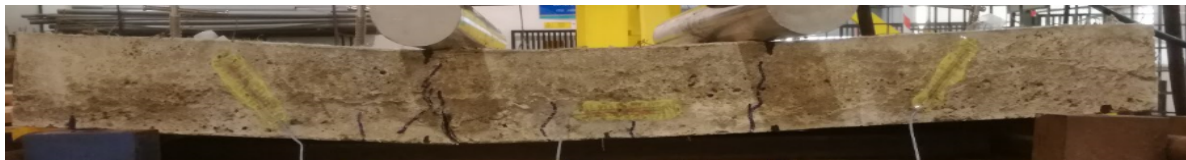
Figure 12. Cracking pattern at the failure of S2-1.
