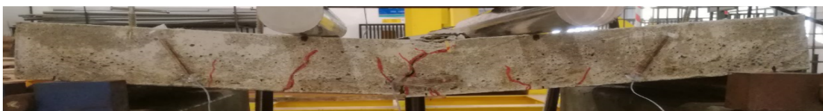
Figure 8. Cracking pattern at the failure of S1-0.
