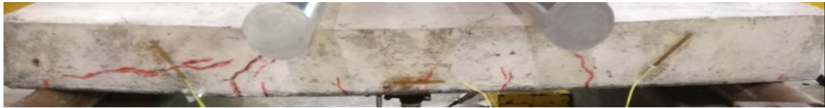
Figure 11. Cracking pattern at the failure of S2-0.
