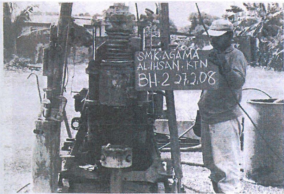
Figure 2.4: Multi-speed rotary wash boring machine (JKR).
