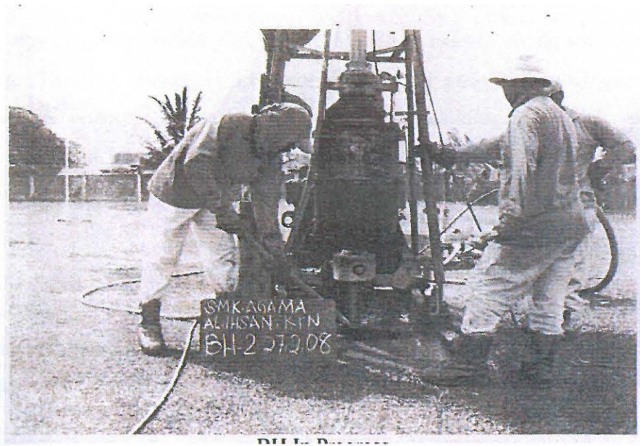
Figure 2.3: Boring work process (JKR).
