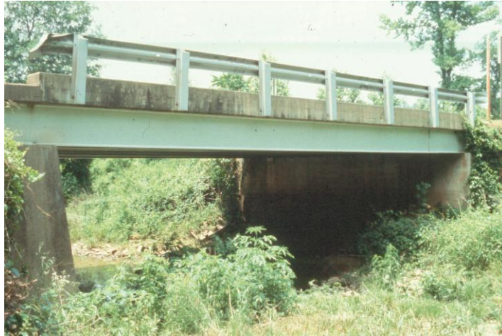
Figure 1.1: Bridge frame using low carbon steel
