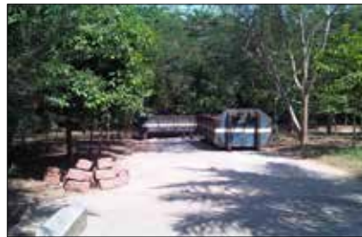
Ash storage facility
