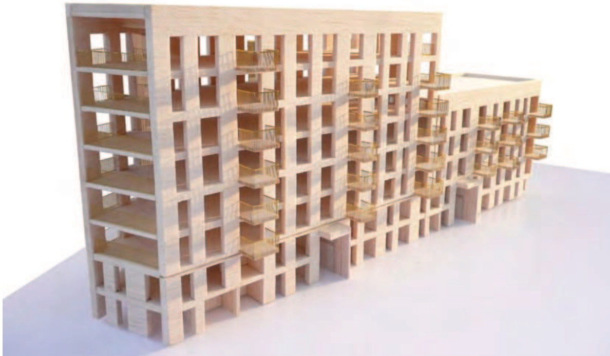
Picture 1 Bridport House CLT frame (Mannevit, S. Karacusevic Carson Architects, Design with Cross Laminated Timber Design and Construction, 2015)
