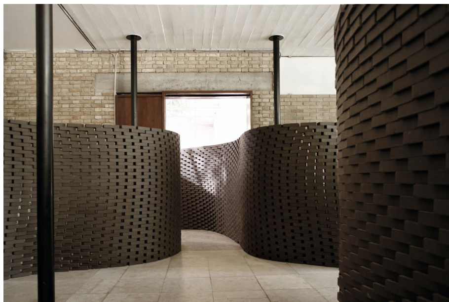
Fig. 3. a, above) Fabrication of wall element. To realize the overhangs a support structure is necessary during the fabrication process; b, below) The completed installation "Structural Oscillation" at the Venice Biennale 2008
