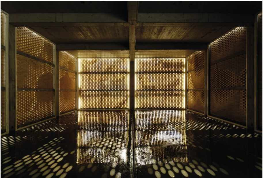
Fig. 4. a, above) A pattern of spheres emerges on the façade of the Gantenbein winery; b, below) View of the interior space illustrating the light atmosphere accomplished through the rotation of the individual bricks
