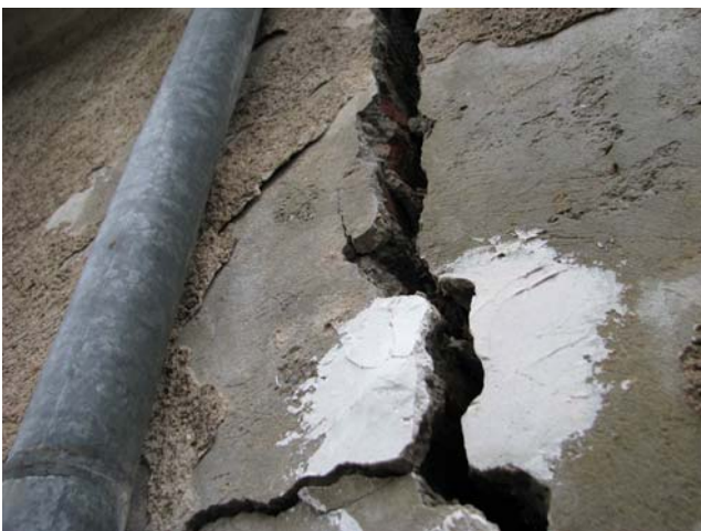
Fig. 2 One of the largest cracks (rainwater gutter for size comparison) in the city centre of Staufen
