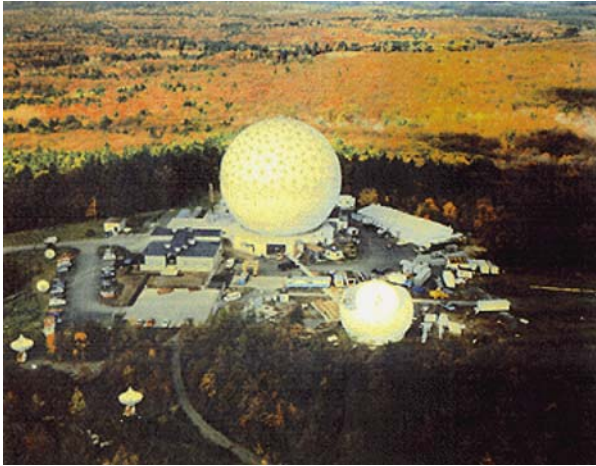
Fig. 10 Haystack radar complex. The 36-m parabolic dish antenna is located under the radome in the center of the figure
