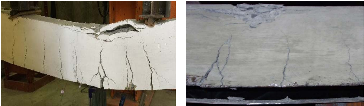
(a) Yielding and crushing of control beams (b) Yielding and crushing of strengthened beams
