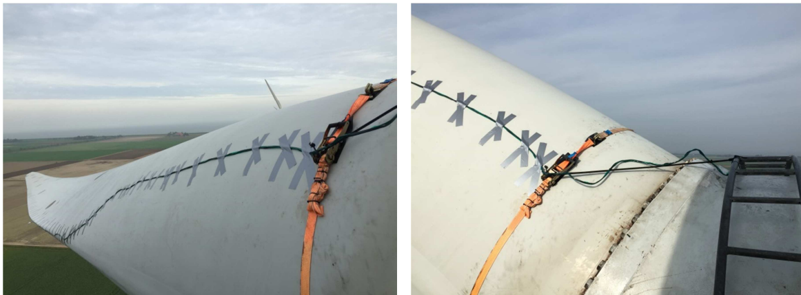
Figure 5. Microphones cabling rooting along the blade
