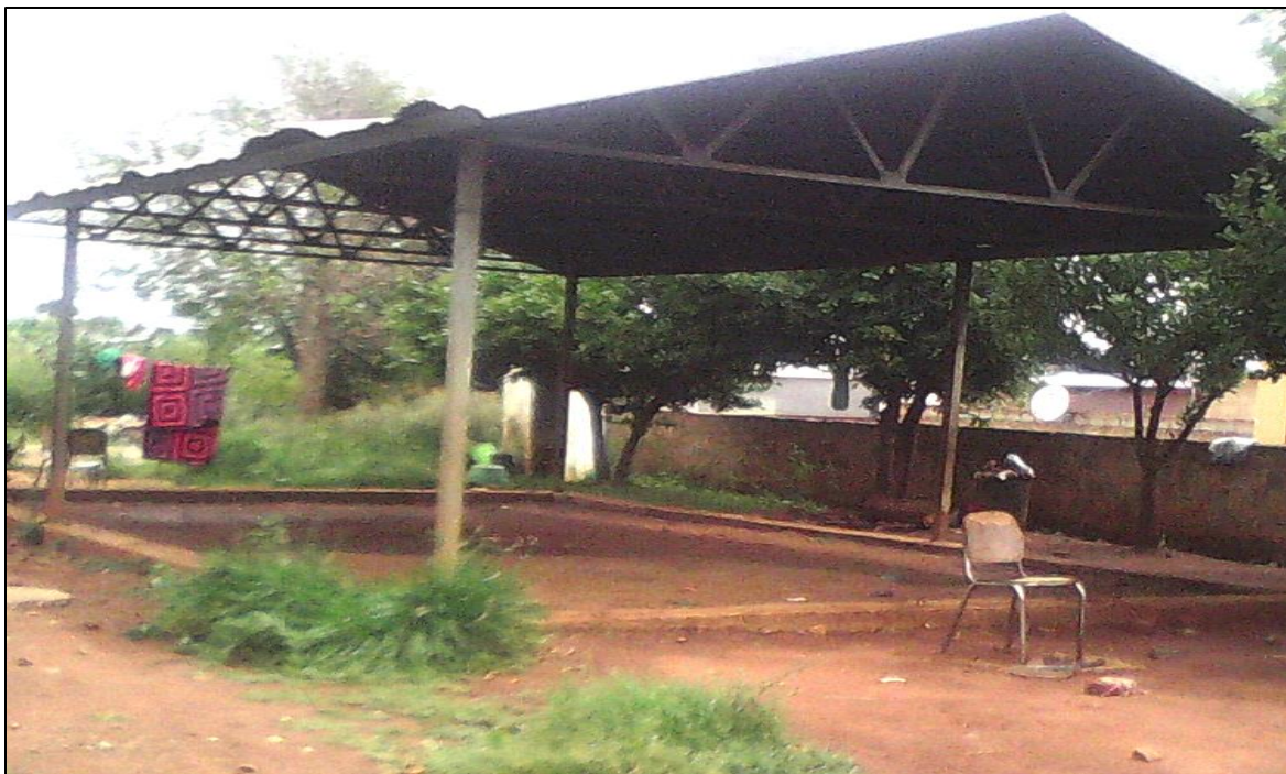
Figure 3.3: Unfinished structure – Example 2
