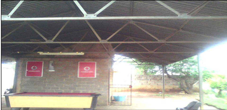
Figure 3.2: Unfinished structure – Example 1
