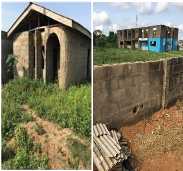
Fig 7: Abandoned building construction projects
