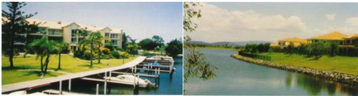
Figure 4: Riverside development is one of the most viable type of river development enable to mitigate river bank from slop-slide
