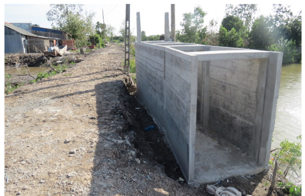
A new sluice gate for shrimp farming under construction
