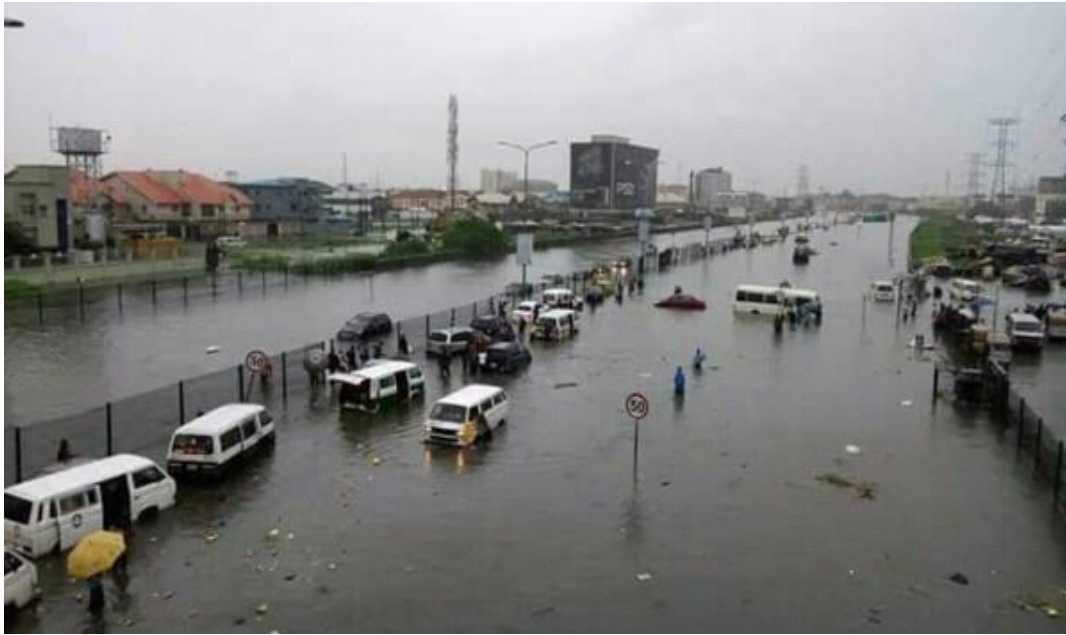
Figure 5: Highway Flood, Lekki Lagos
