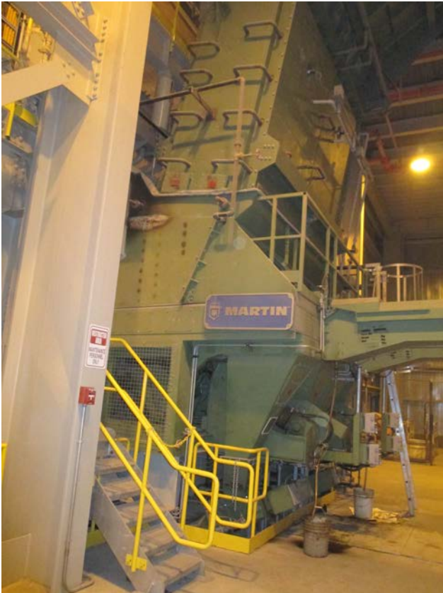
Fig 1.6 – Martin Grate System Boiler
