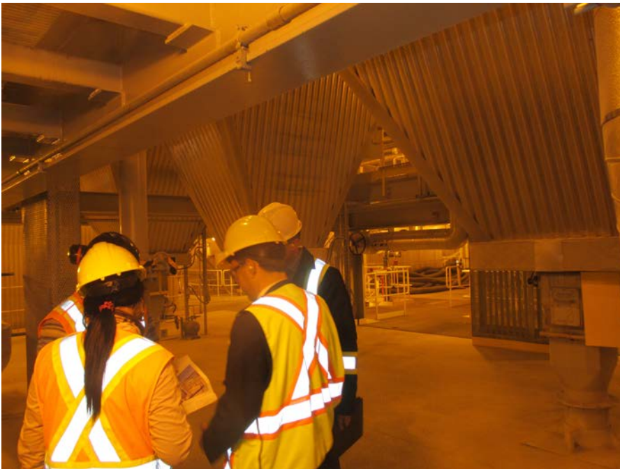
Fig 1.10 – Fly Ash Hoppers
