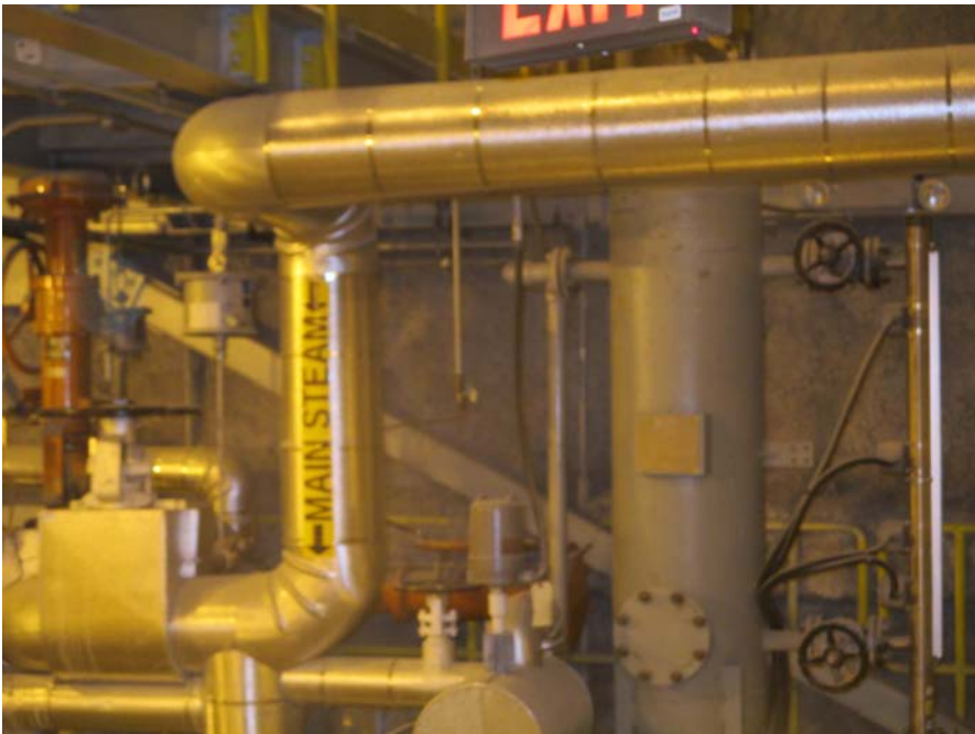
Fig 1.12 – Pipes Sending Steam To Generators
