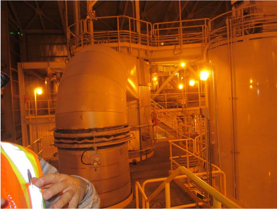
Fig 1.10 – Fly Ash Hoppers
