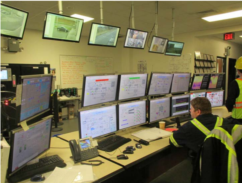
Fig 1.4 – Incinerator Control and Emission Monitoring Centre
