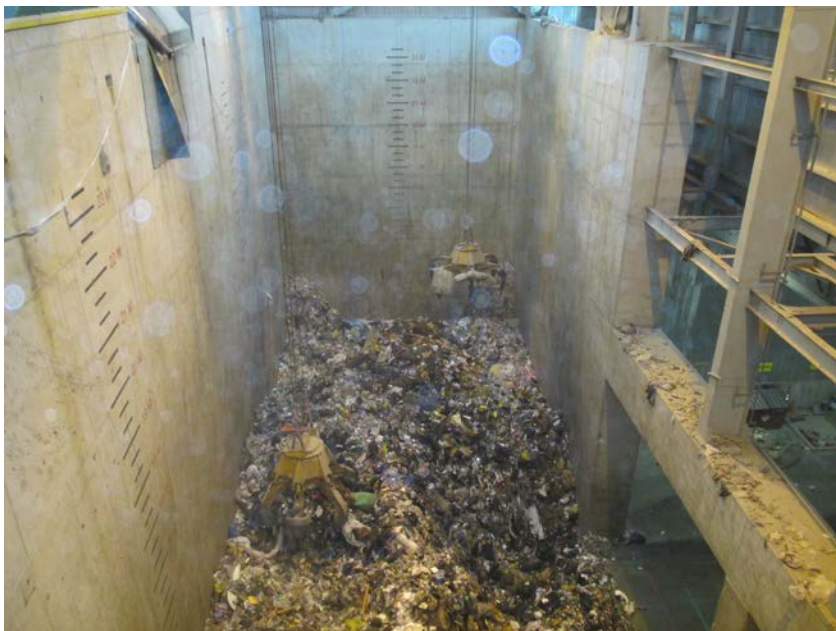
Fig 1.2 – Tipping Floor and Feeder
