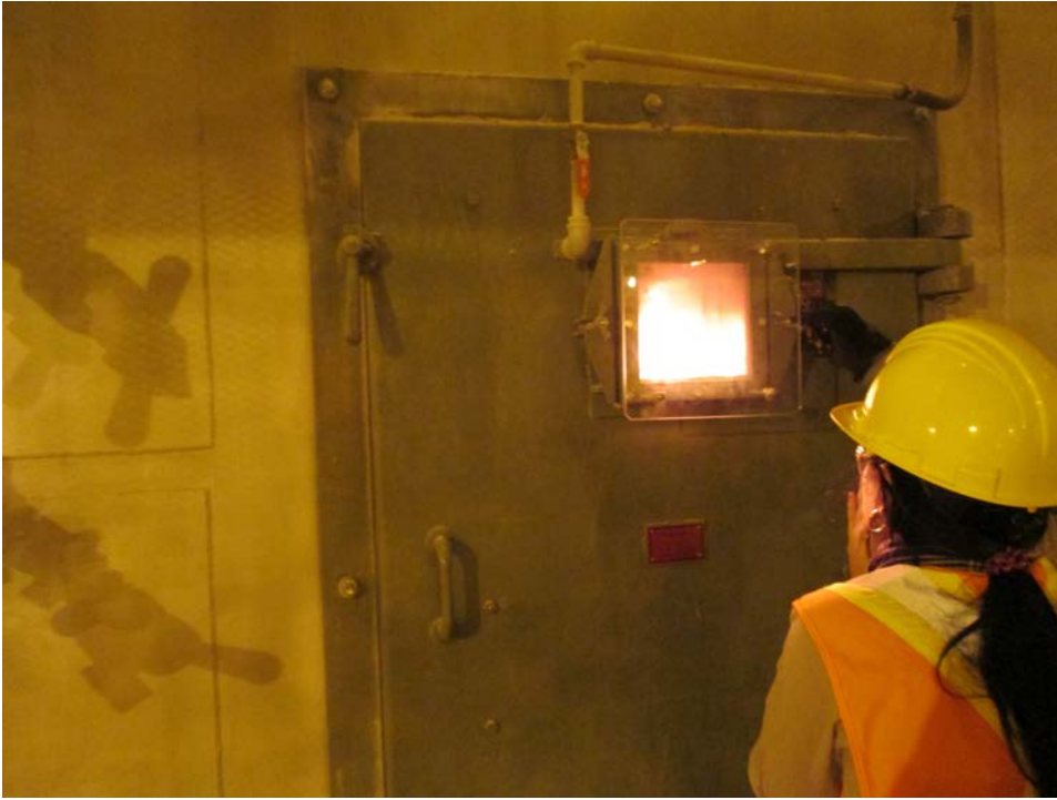
Fig 1.8 – Bottom Ash Expeller
