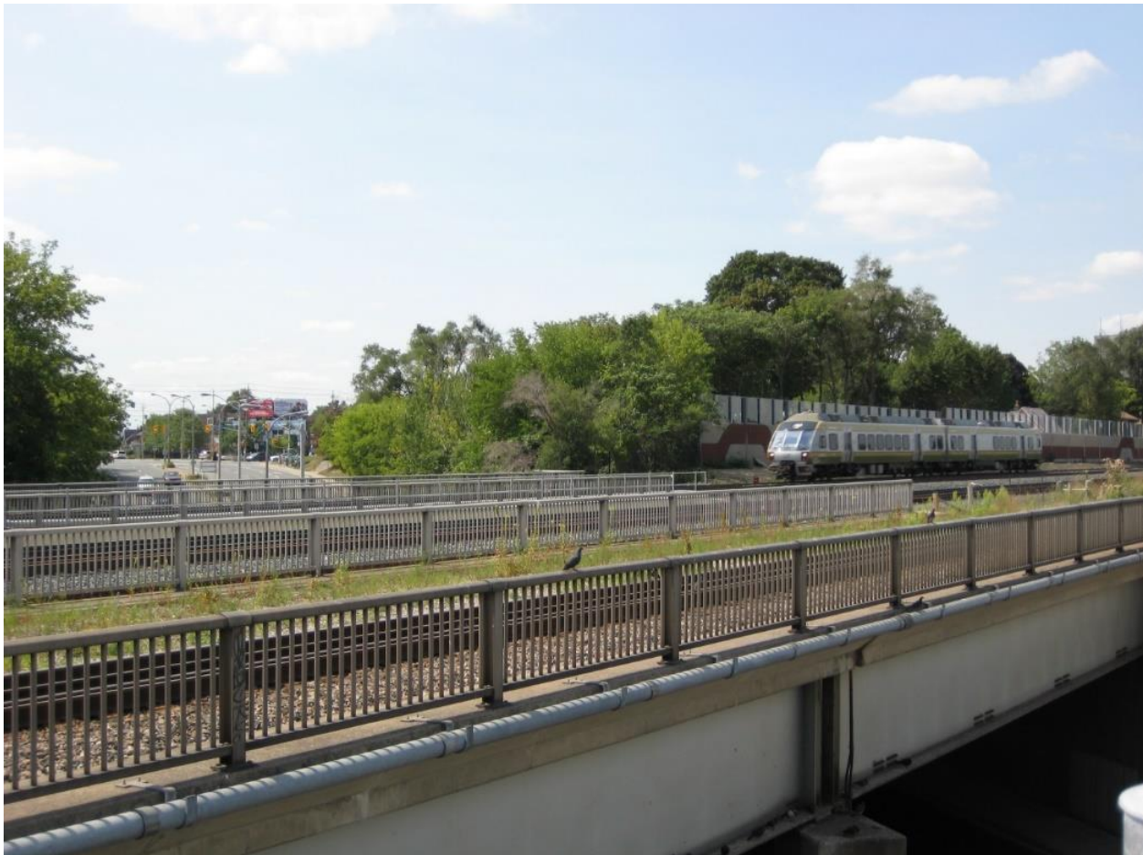
Figure 28. Metrolinx rail overpass (Kitchener Line) at Eglinton Avenue West, looking west, Mount Dennis, York, Ontario. The Union-Pearson Express may stop here in the future with an interchange to the Eglinton Crosstown line. Source: Michael Collens.
