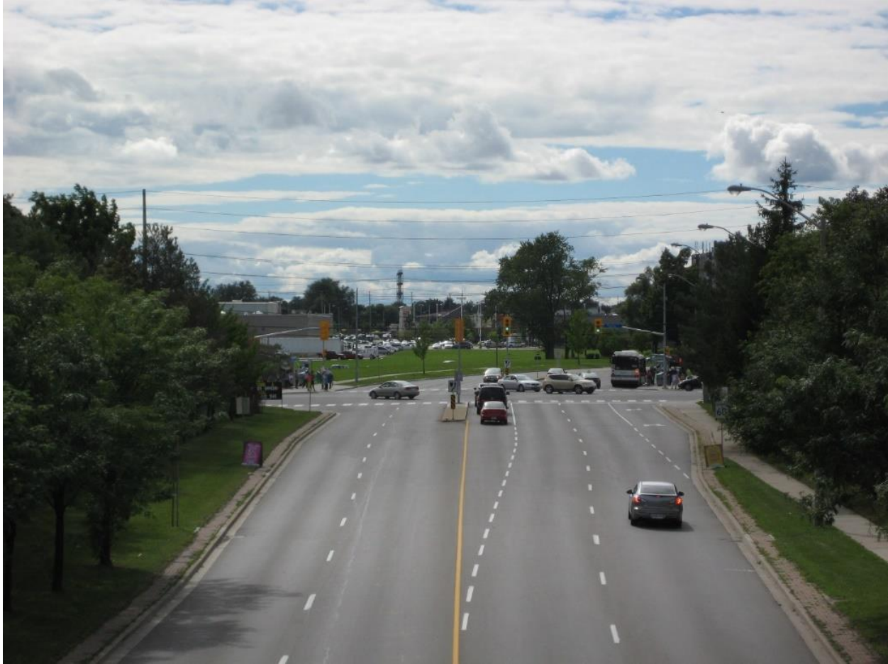
Figure 33. Finch Avenue West, looking west towards Kipling Avenue, Mount Olive, Etobicoke, Ontario. Wider road lanes with turning lanes at the intersections make the roadway more difficult to navigate for children, seniors and persons with disabilities by extending the distances they need to travel and exposing them to more lanes of traffic. Source: Michael Collens.
