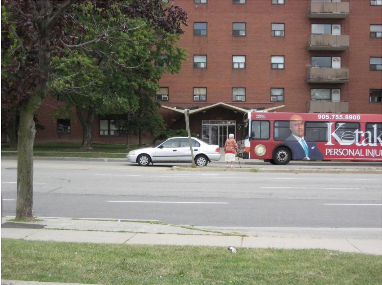
Figure 20. Bloor Street, east of Dixie Road, Applewood, Mississauga, Ontario. Poor pedestrian access to the residential buildings from High Point Mall (background). Source: Michael Collens.
