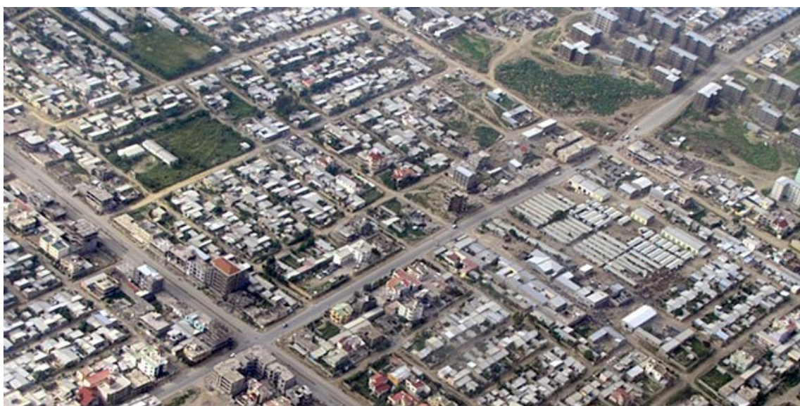
An aerial view of Mek'ele, the capital city of the Tigray region of Ethiopia
