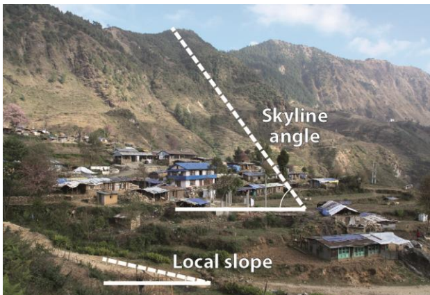
Figure 1. Landslide-prone houses in Sindhupalchok District, Nepal, showing the difference between the maximum angle to the skyline and the local slope of the ground surface.
