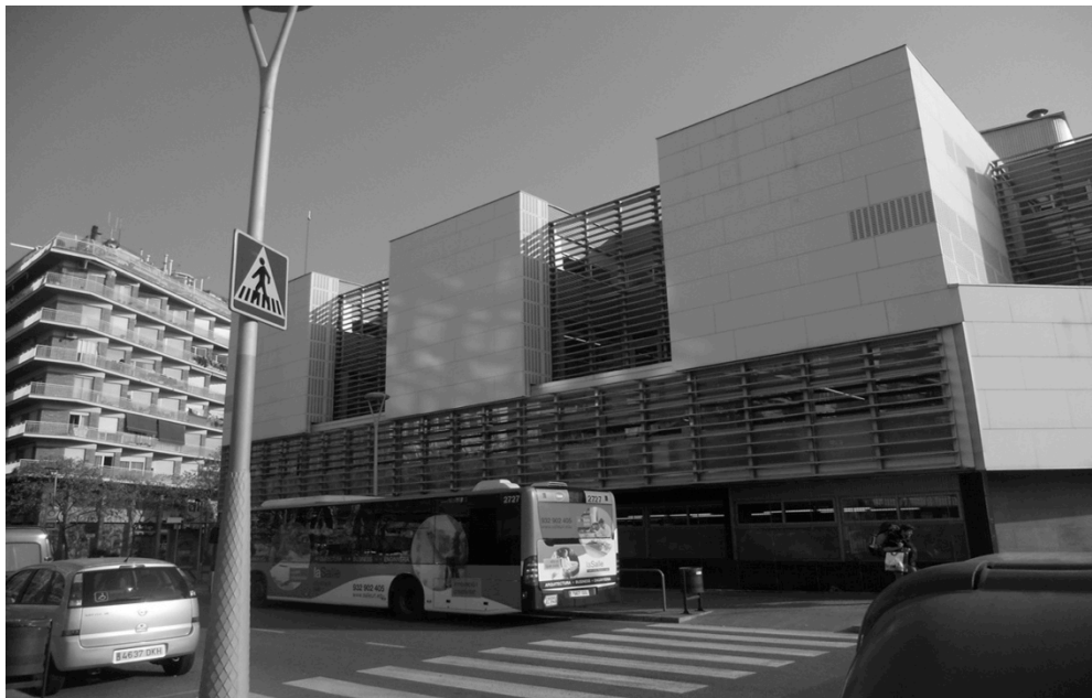
Figure 13. Façade with unmovable blinds with a bus station in front (Source: Pupils, 2012)
