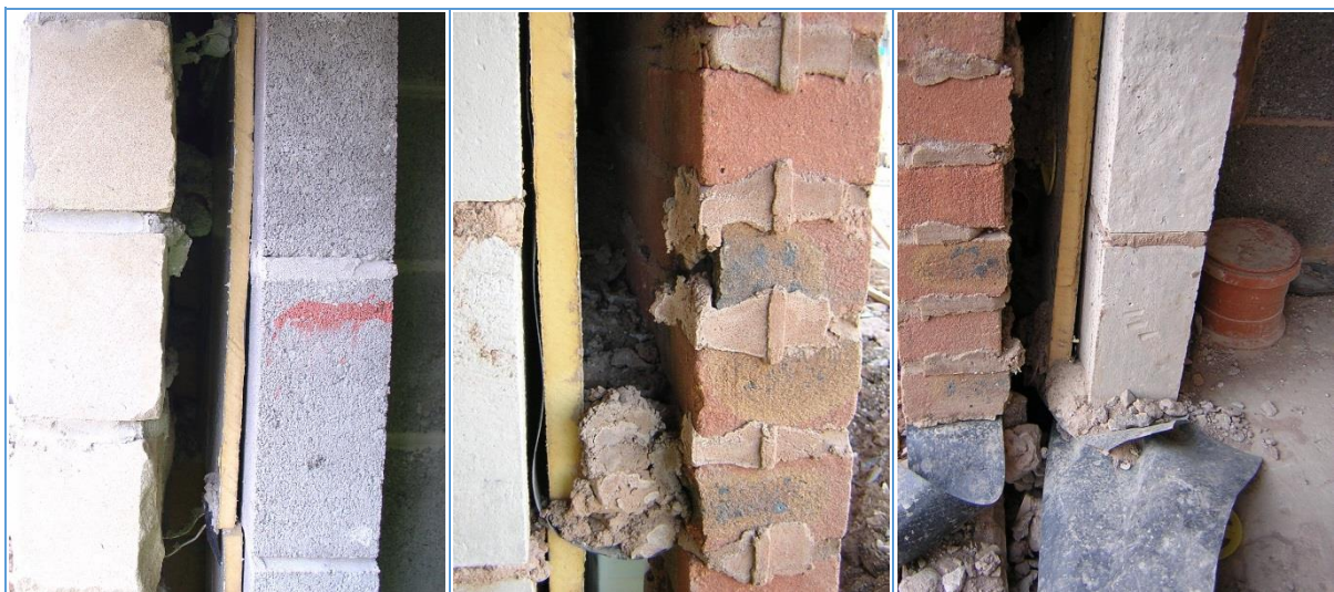
Figure 21 Partial-fill boards are not positioned flush with the inner leaf blockwork
