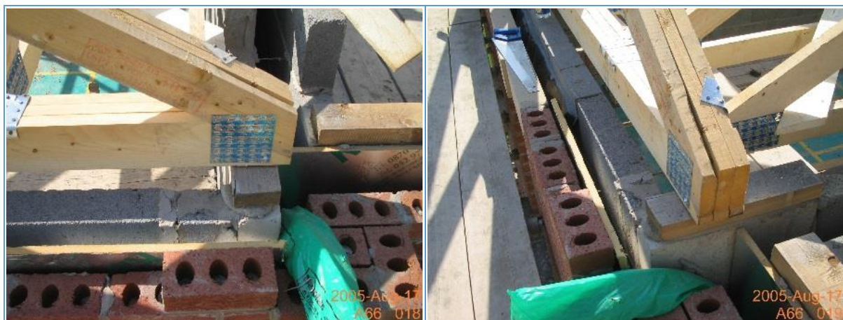
Figure 29 Staggers and other more complex junctions
