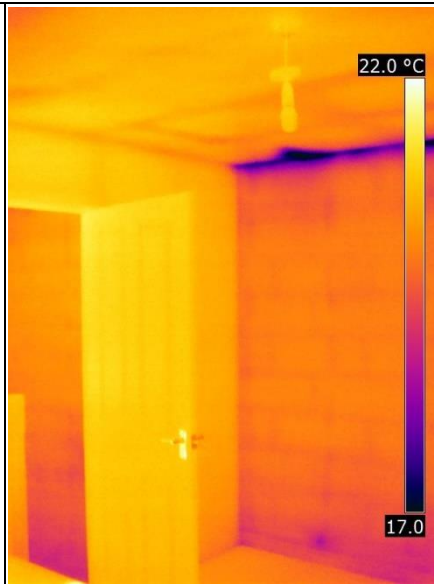
As observed in bedroom 2.
