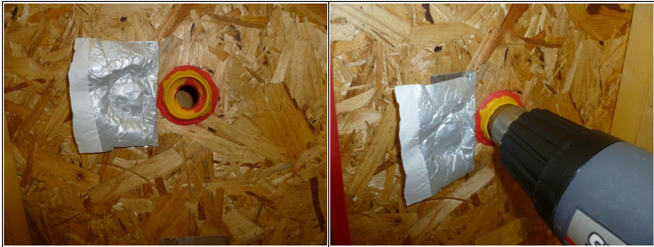
Figure 6 Forced air injection point and seal
