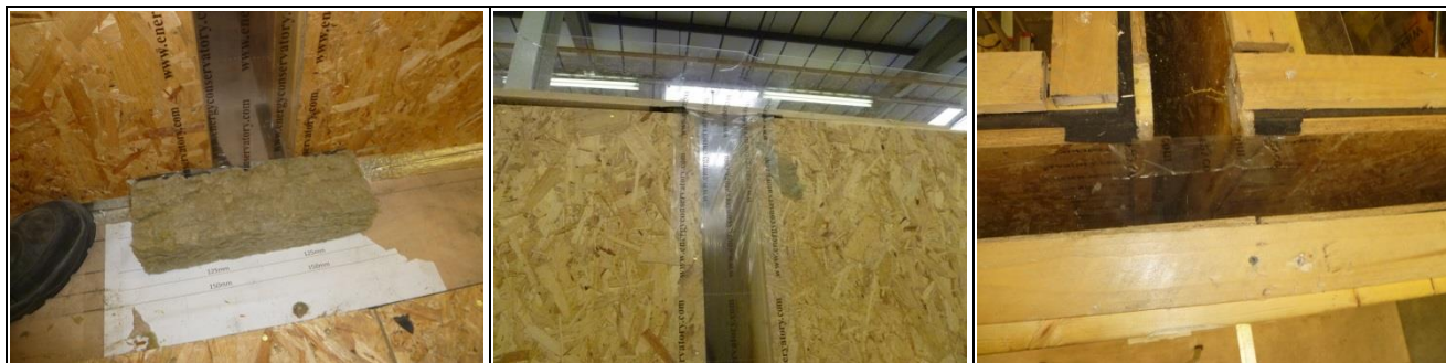
Figure 60 Test 4.18, DuctMask™, 100 mm party wall, 100 mm external wall
