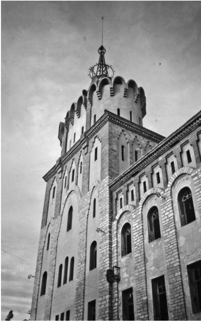
FIGURE 9. Flour mill of the Sindicat Agrícola of Cervera and its county. Close-up of the façade and the water reservoir. Photo: R. Lacuesta, 2012.
