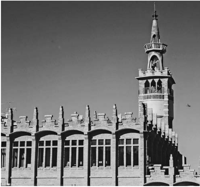
FIGURE 3. Close-up of the Casaramona factory with one of the towers housing the water tanks. Photo: Ramon Manent.
