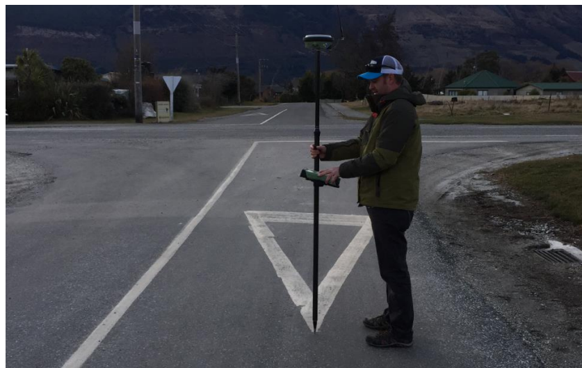
Figure 6.14 Collection of RTK measurement of a road marking within the township of Glenorchy to provide extra independent control points.
