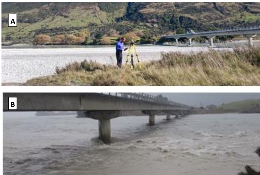
Figure 3.2 Both images taken two days apart from opposing sides of the Bridge at the Hillocks, (A) a low flow of \sim 50 \text{ m}^3 \text{ s}^{-1} and (B) a peak flow of \sim 700 \text{ m}^3 \text{ s}^{-1} .
