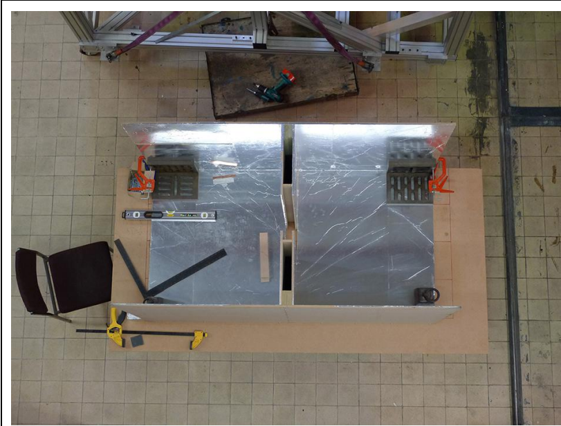
Building the anechoic chamber.
