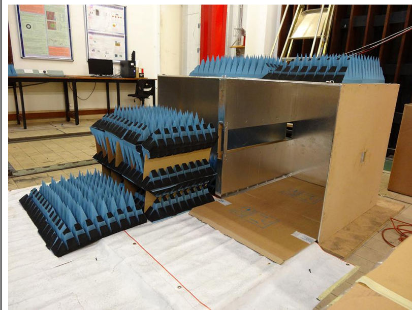
Building the anechoic chamber.
