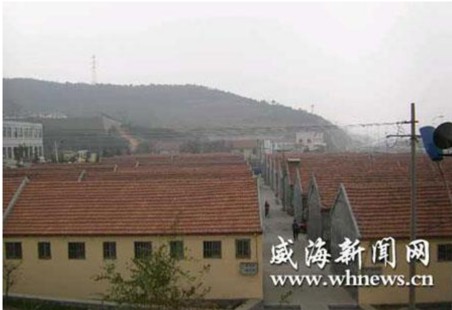
Picture 19 Temporary Living Houses During Redevelopment Construction Period
