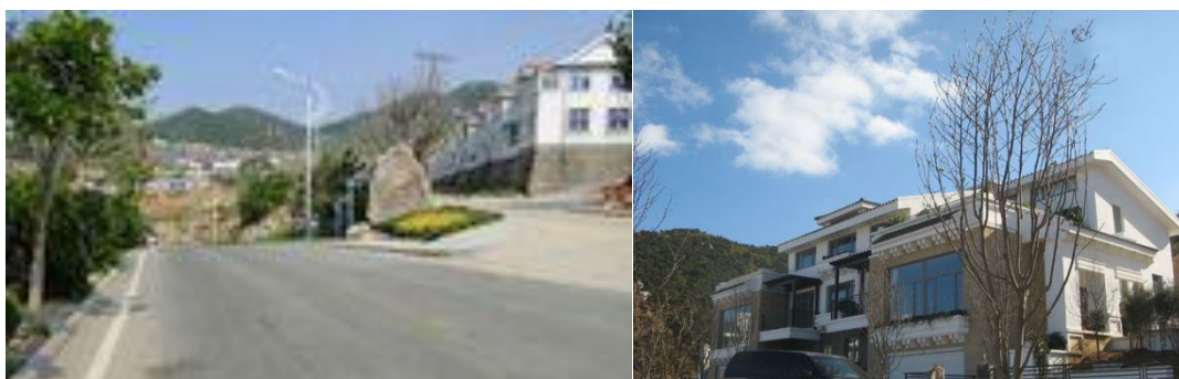
Picture 24 New Built Houses Outside Features Li Yao
