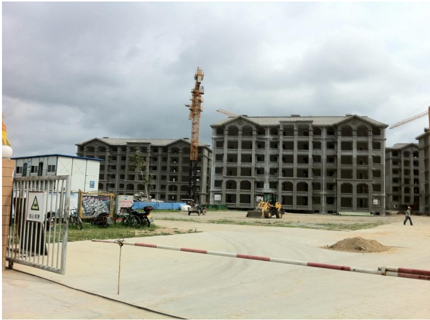
Picture 12 Construction of Wen Quan Tang New Residential Building
