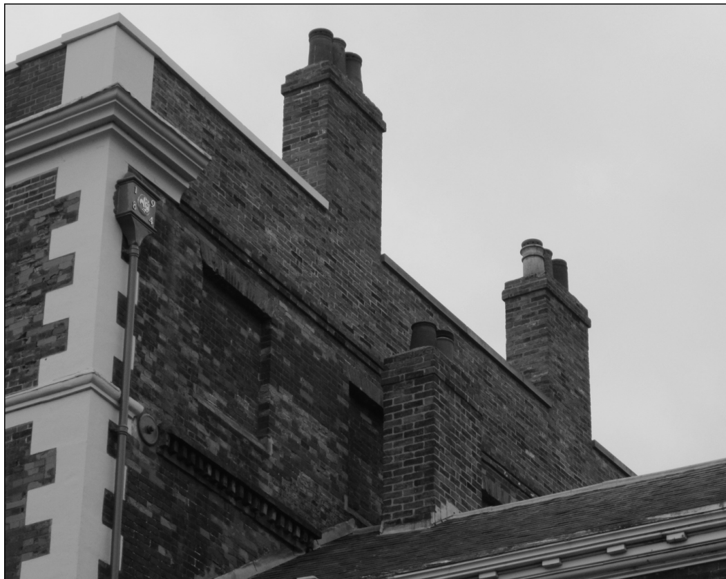
Figure 1.6. View of the south-eastern end wall of Fairfax House, showing blind window openings and remains of original ornamental band and cornice. (Author's picture, October 2015.)
