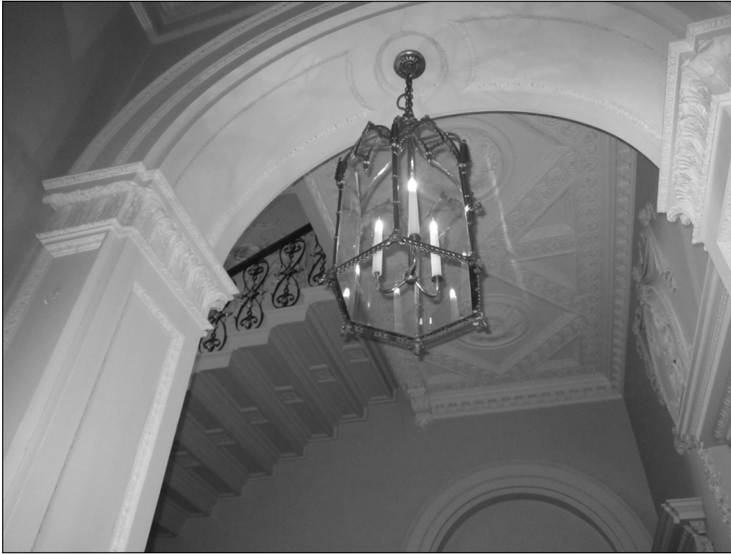
Figure 1.13. View into the Staircase Hall from the Entrance Hall, showing the elaborate plasterwork beneath the first-floor landing of the Great Staircase. (Author's photograph, 2014.)
