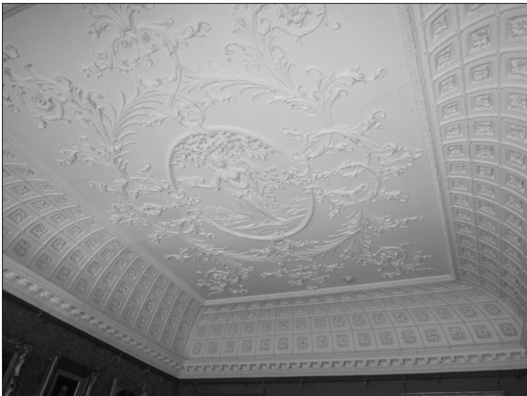
Figure 1.21. The ceiling of the Drawing Room, showing the deep coving with coffered decoration and the central figure of 'Amicitia'. (Author's photograph, 2015.)
