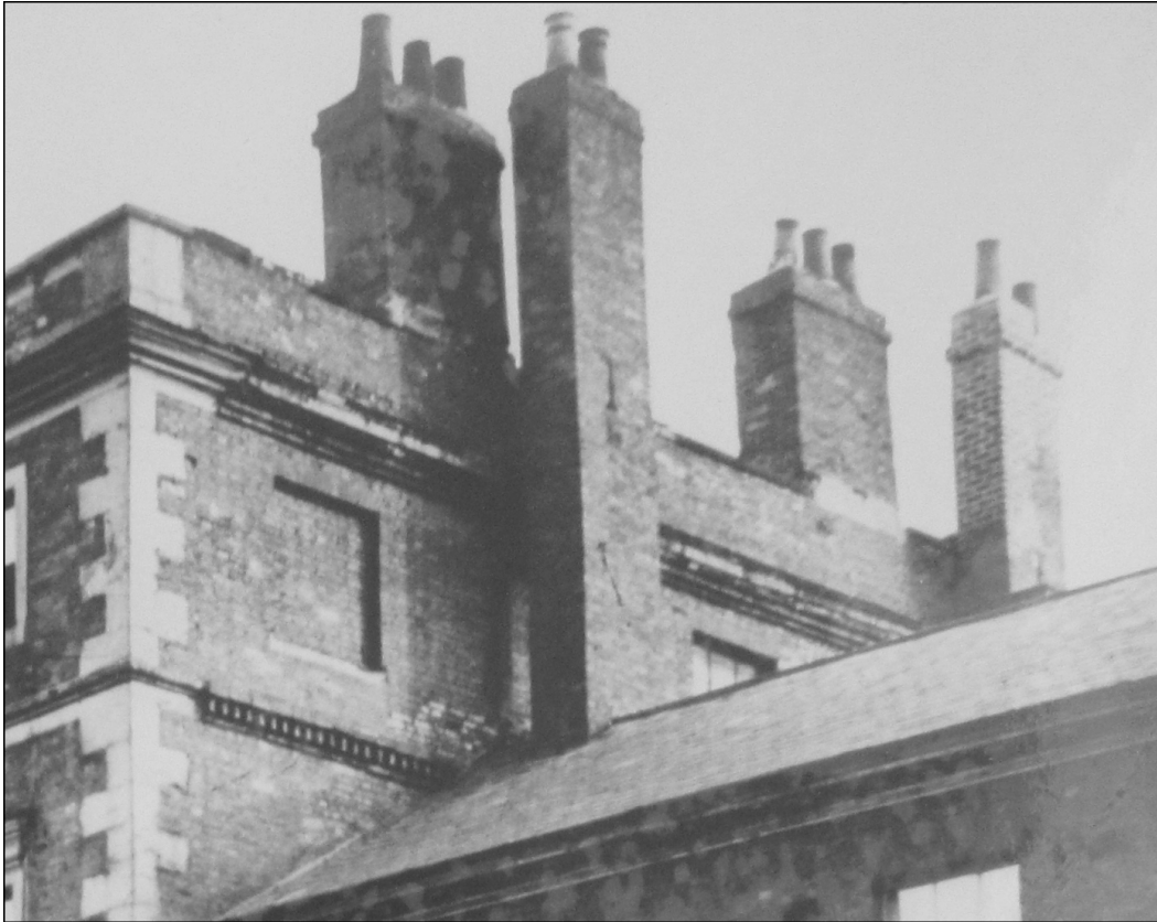
Figure 1.7. Detail of photograph of Fairfax House taken c.1900, showing glazed window opening in south-eastern end wall. The original decorative cornice on this wall is also visible. (Fairfax House Archives.)
