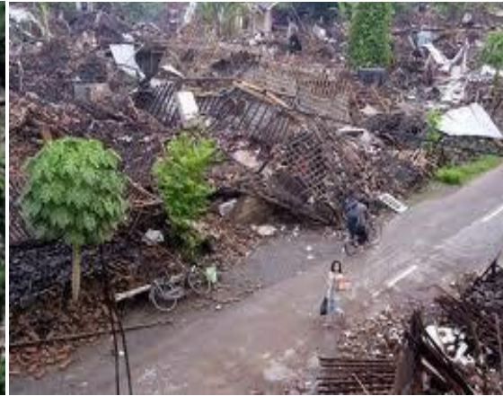
Houses damages from Bantul earthquake
