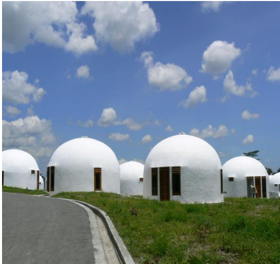
Dome House construction
