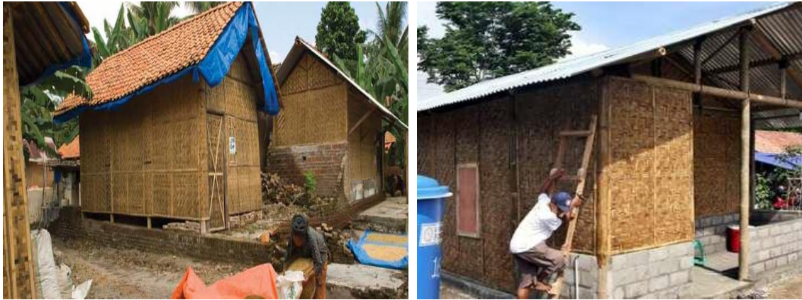
Figure 8.4 Transitional shelters at Sleman district (Source: JRF, 2011)
