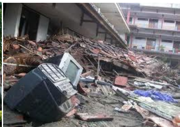
School building damages from Bantul earthquake
