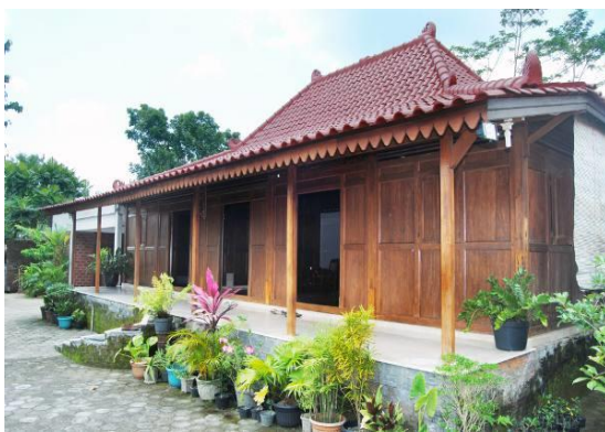
Original Javanese house with most of parts constructed by woods/bamboos with high roof and many windows to adapt with high temperature
