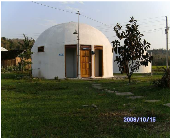
EcoShells that include laundry, toilet and shower facilities, were constructed. Each was placed between two neighboring clusters of dome-homes.
