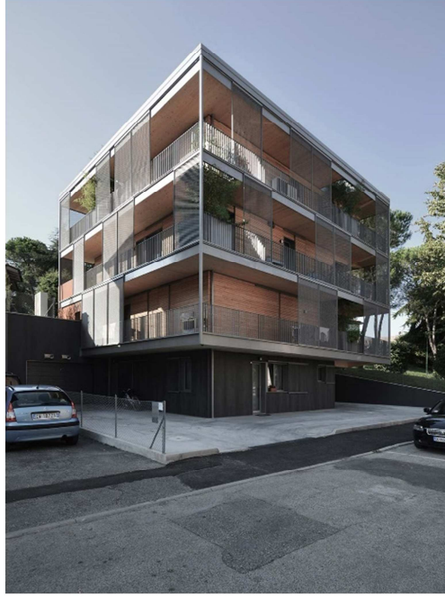
Figure 1. Outdoor view of the Fiorita passive house
