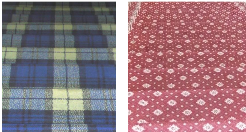
Figure 2.4 Patterned carpets obscuring stair edges
