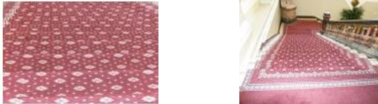
Figure 3. Stair edge obscuration due to patterned carpet.
