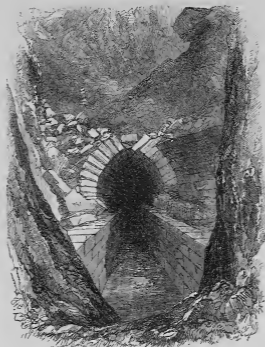
Vaulted Drain beneath South-east Palace (Nimroud).
