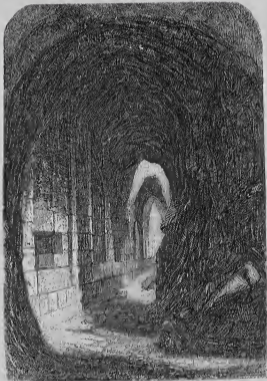
Tunnel along Western Basement Wall (Nimrud)
