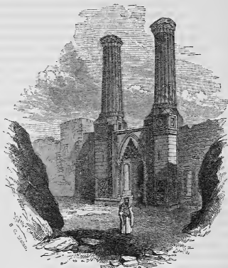
Ruined Mosque and Minarets (Breastroom).
