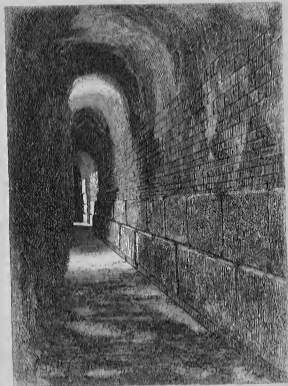
Tunnel along Eastern Basement Wall (Nimrud).
