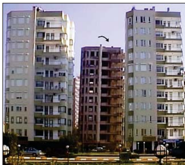
Figure 1. Leaning apartment building in Antalya (Turkey).
