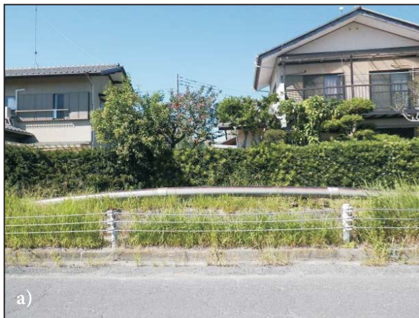
Figure 15. Uplift of (a) pipeline in reclaimed land of Itako city and (b) underground tank in Kozaki town.
