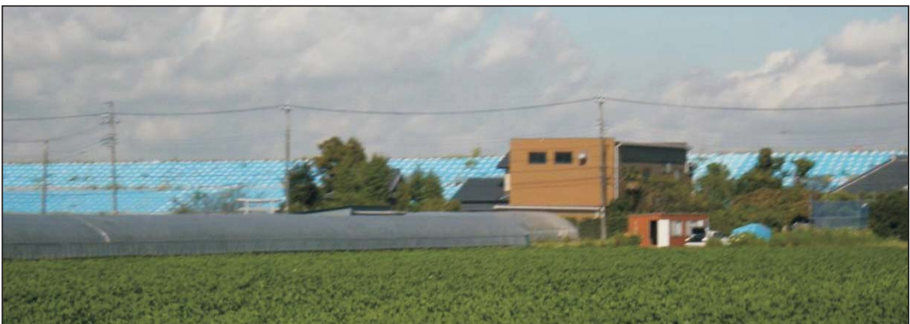
Figure 13. Extensive protection of the damaged Tone river dike (Sakae town) against rainfall.
