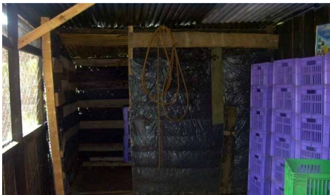
Plate 2. Charcoal cooler on farm in Yatta.
