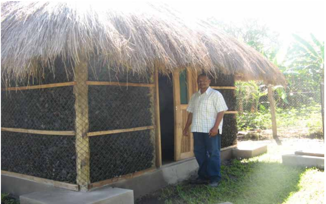
Figure 2. A charcoal cooler at Sulma foods in Luwero, Uganda.
