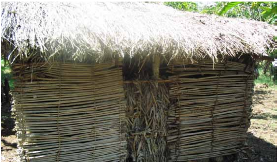
Figure 1. Cooling shed made out of local materials at one of the vegetable farms in Wakiso, Uganda.
