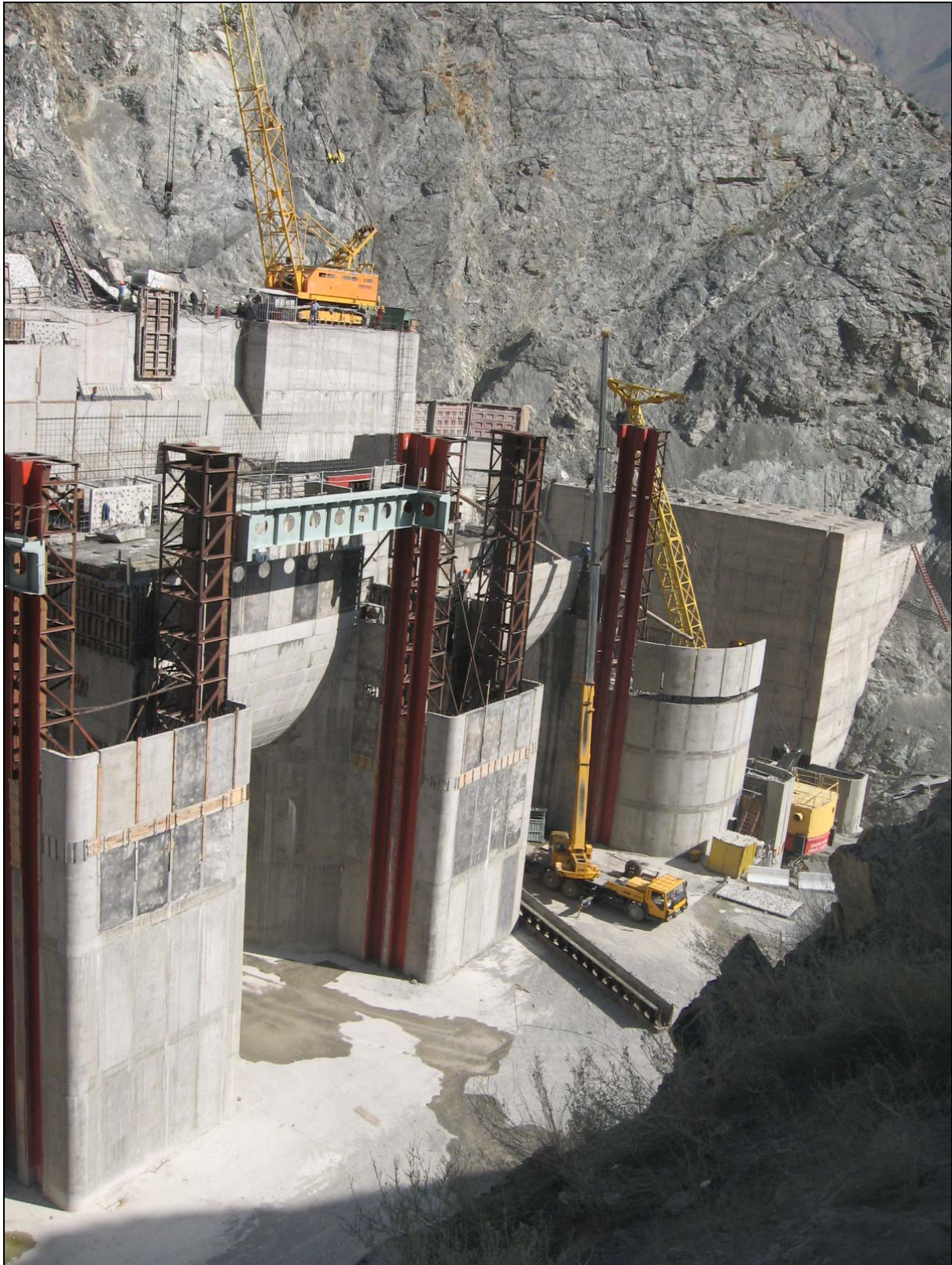
Figure 13: Construction work on Kamar Ata 2 dam in 2009
