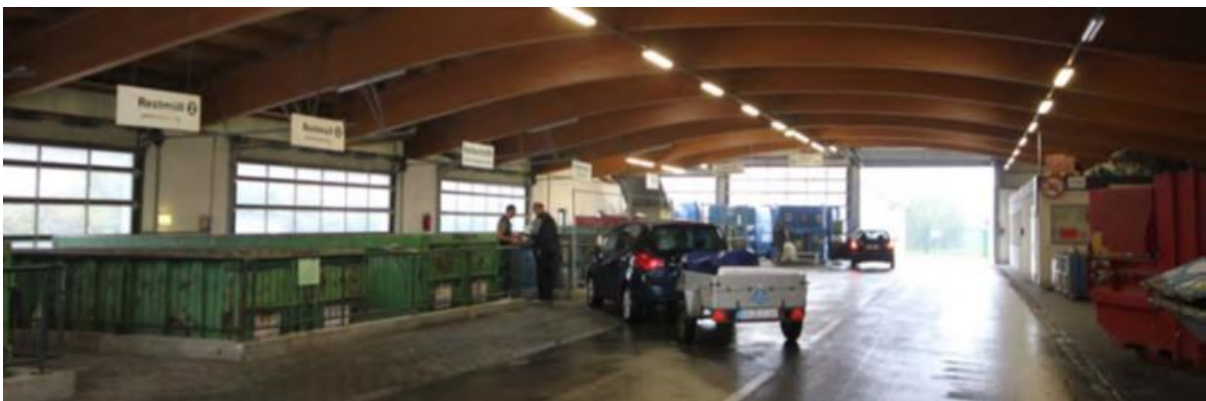
Figure 4-42. Example of a roofed collection centre (ia GmbH / UMSICHT, 2015b, p 17)
