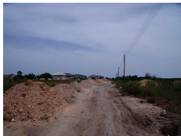
Encroachment into the wetland south of Tetegu
