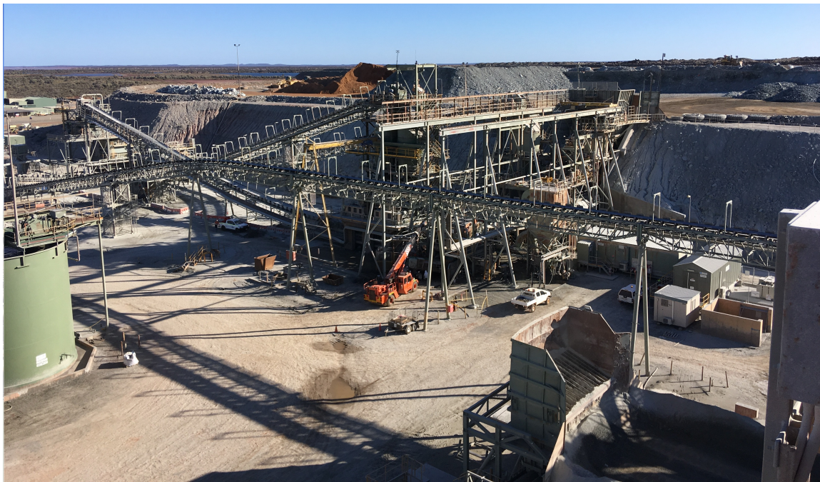
Figure 6.2: ROM pad with primary and secondary crushers and additional conveyor belts at SDGM.
