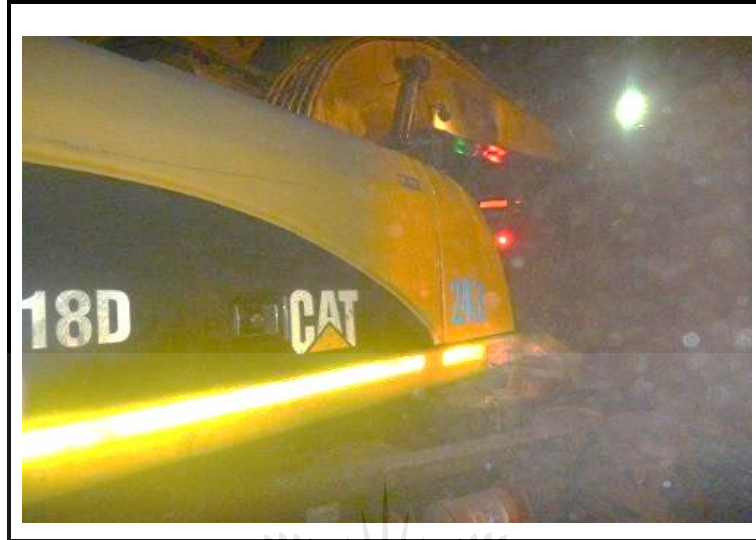
Figure 33: Track excavator operating at the mining section
