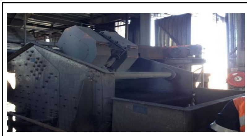
Figure 38: Second floor screen
