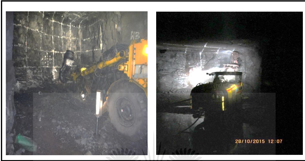
Figure 35: Double boom drill rig operating
