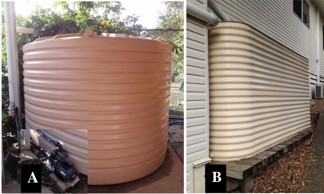
Figure 7. Modern circular design 10,000L rainwater tank with electric pump and first flush diverter (both to the left side)(A). Slimline 3,000L rainwater tank designed to fit into smaller spaces (B).
