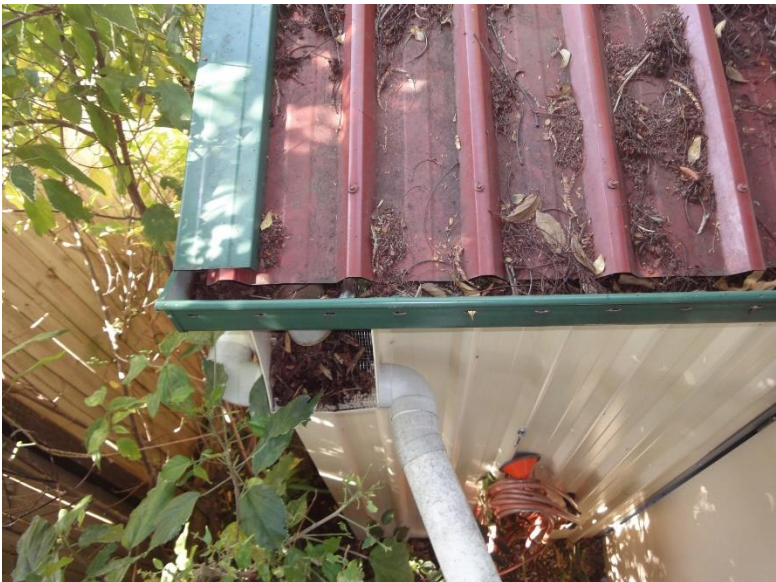
A9. Gutters observed that likely increased productivity of rainwater tanks in Brisbane and Gin Gin, 2014.
