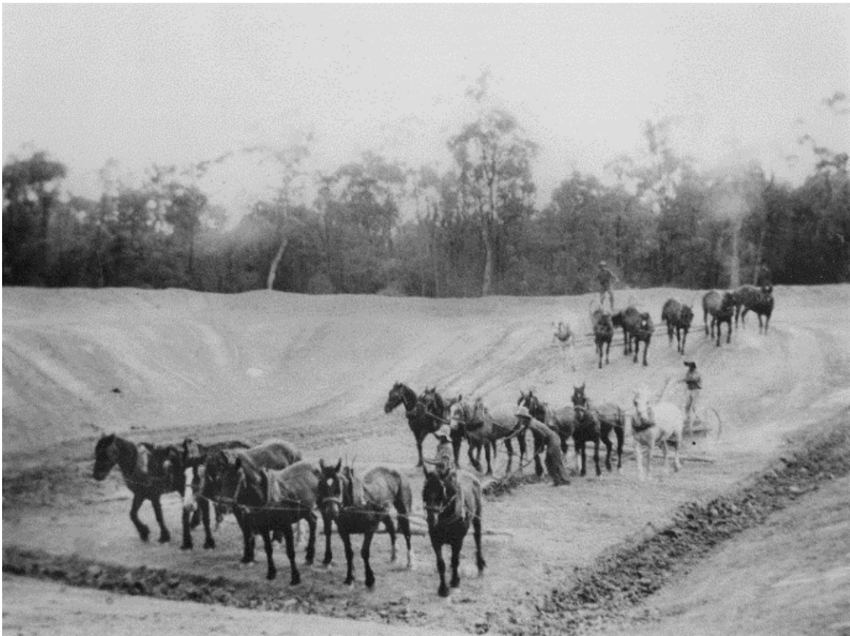
Image 5 Water management: Horse teams and ploughs used to dig dams, Tara district 1932 (source: SLQ)
