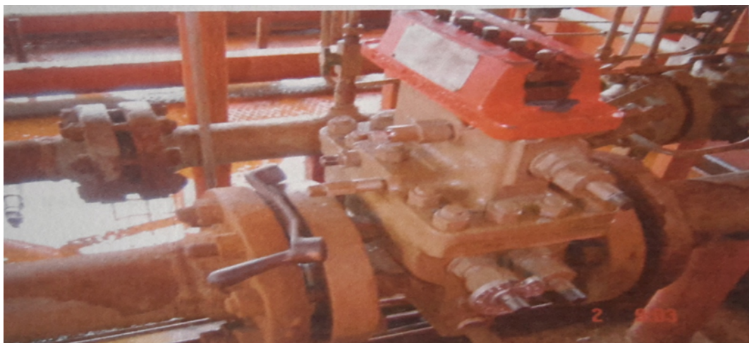
Figure 3: Gas orifice metering system.
