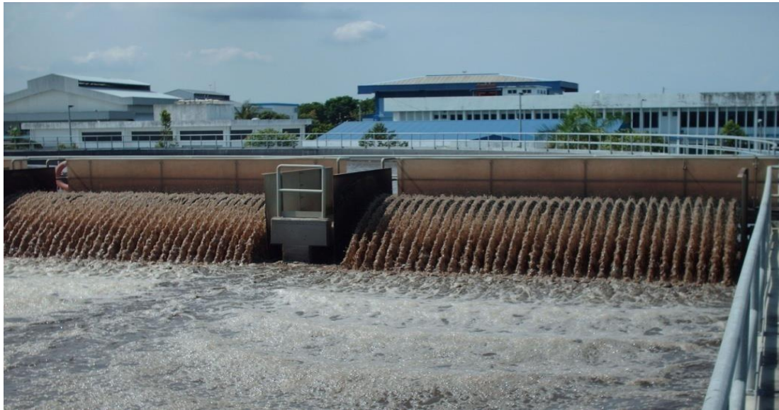
Figure 3.11: Rotating discs as mechanical aeration devices
