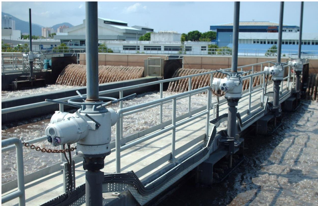
Figure 3.12: Four penstocks gate between channels
