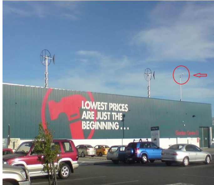
Figure 4- Position of the ultrasonic anemometer on the roof of the Bunnings warehouse.
