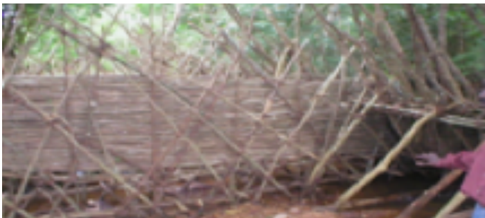
Plate 14. A strong fish fence across a stream with high currents in which sticks are used to strengthen the structure.
