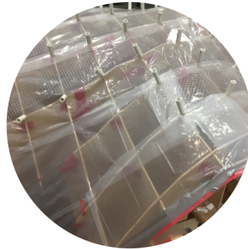
POLYETHYLENE PLASTIC IS USED AS WATER BARRIER
